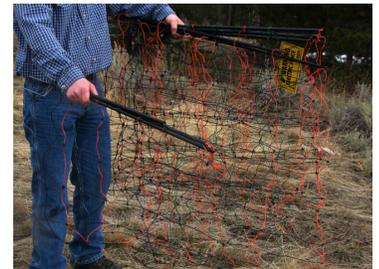
2. Push post #1 into the ground at your starting point. This fence has a positive/negative configuration. This is the safest type of fence for bears. It insures a ground connection and does not depend only on the earth ground. One of the end posts has extra separation tubes for the Pos/Neg configuration. This is post #1.
